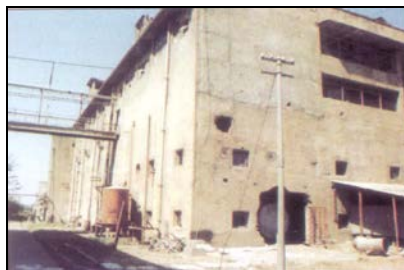
Photograph - A shows the building in which aluminium trays are installed. The building is specially designed with walls having abnormally high thickness (1000 mm) with height of about 15000 mm and a large built-up area.
