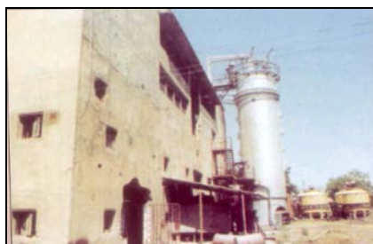
Photograph - A shows the building in which aluminium trays are installed. The building is specially designed with walls having abnormally high thickness (1000 mm) with height of about 15000 mm and a large built-up area.
